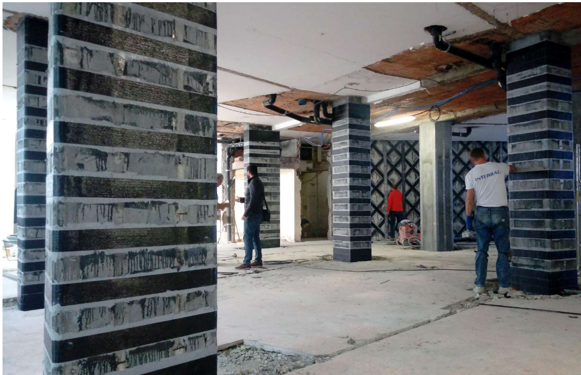
2017 SEISMIC RETROFIT G.F.L. - LA MADONNINA HOSPITAL MILAN
